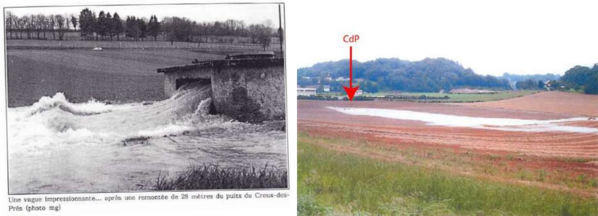
Figure 6—7. Right: overflow of CdP during the flood event of April 4<sup>th</sup>, 1992. The supposed discharge rate on the picture is about 3 m<sup>3</sup>/s, even more (Maurice [1993]). Left: overflow of CdP during the flood event of August 2007 (9<sup>th</sup>); order of magnitude of the estimated peak discharge rate was about 2 to 4 m<sup>3</sup>/s (picture from J.-C Bouvier)
