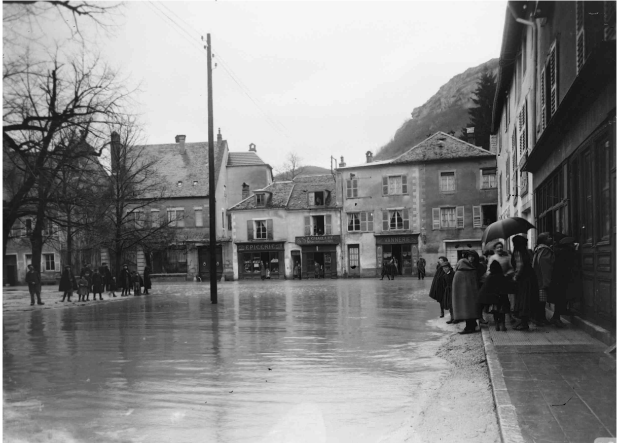
Inondations place Courbet
