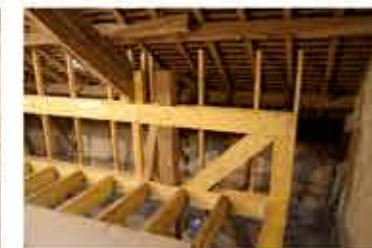
Structure poteau/poutre treillis
